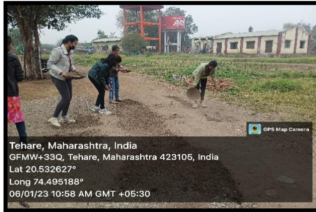
NSS volunteers repairing road at Tehere
